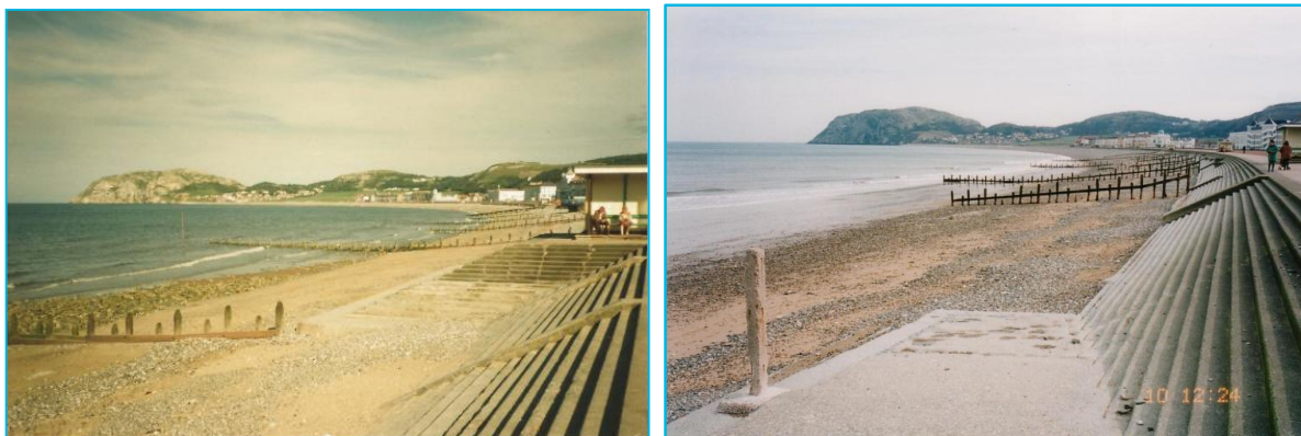
Figure 2.4 – Stepped Revetment, Beach and Groynes 1987 (left) and 1995 (right)
