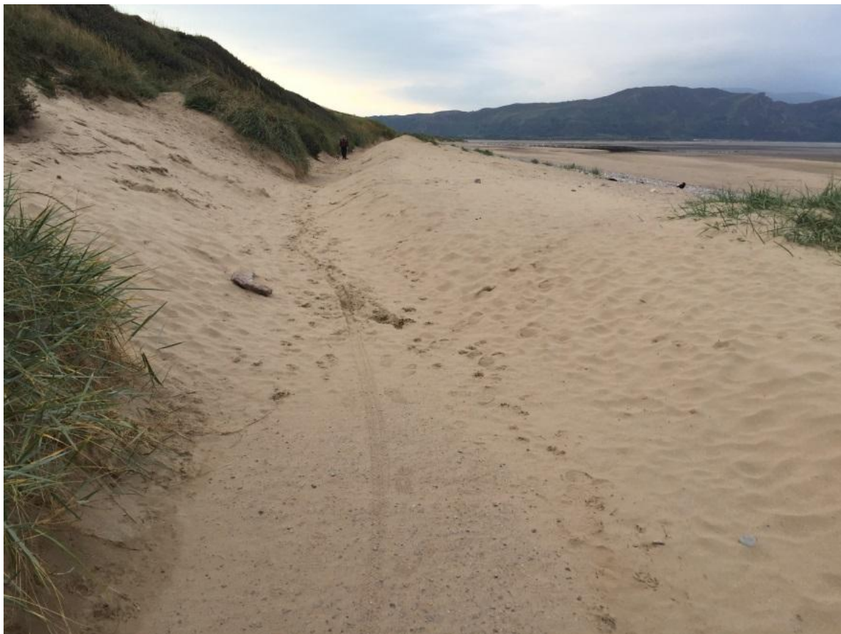
Figure 3-3. Build-up of material along the West Shore cycle path (AECOM, 2016)
