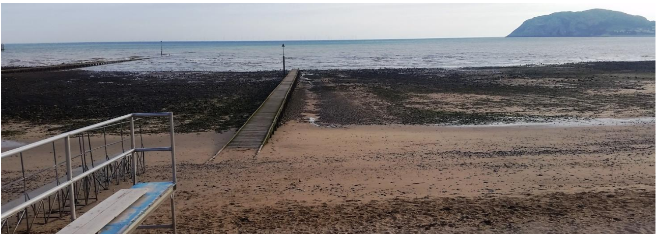
Photo 5 Timber slip way with little evidence of any interruption of drift sediment transport.
