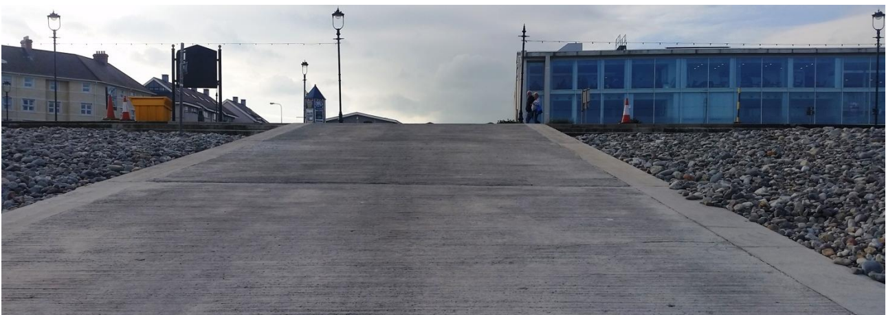
Photo 5 Existing concrete slip way.
