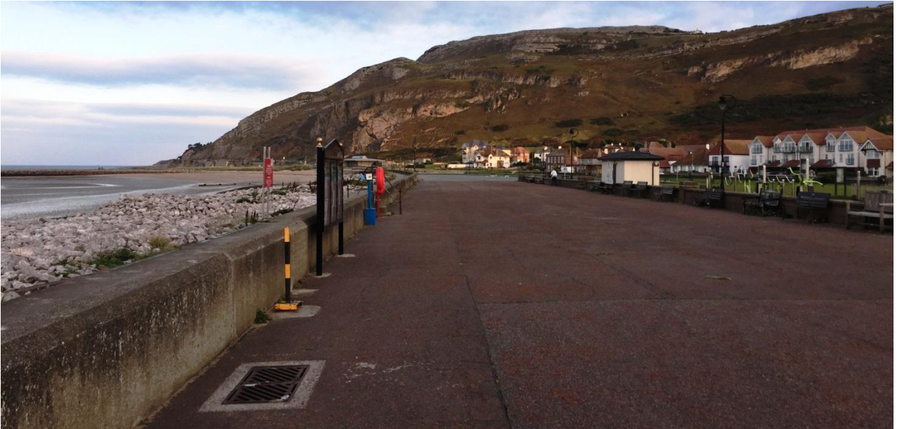
Photo 12 Existing flood wall (with excess sand on the landward side in places), promenade, recreational open space with outdoor exercise equipment and sea fronting residential properties.
